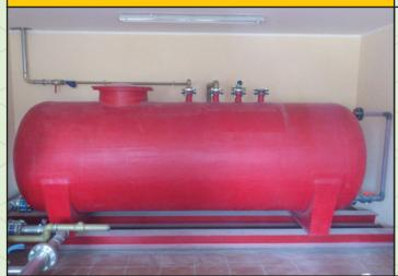
In this system, compressed air is stored separately to be mixed with water only at the time of activation. When the system gets activated, water and compressed air mix together from two different sources to spray Watermist through the specialized nozzle.
