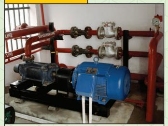
A large area where higher quantities of Watermist may be required to curb a fire needs a bigger source of water. In such cases, the water is stored in a local tank/reservoir which is connected to a pump and in the event of a fire, the high-powered pump propels water from the reservoir/tank efficiently to the pipes and specially designed nozzles.
