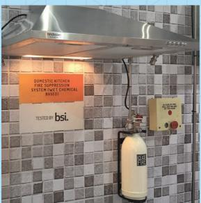
The Wet Chemical based kitchen fire suppression system is ideal to fight Class A, B and fires arising in the kitchen. Wet chemical has a blanketing effect on the flames which cool the super heated oil to below its self-ignition point bringing the fire in control.
